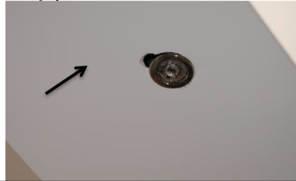
Hole by Sprinkler in Multipurpose Room
