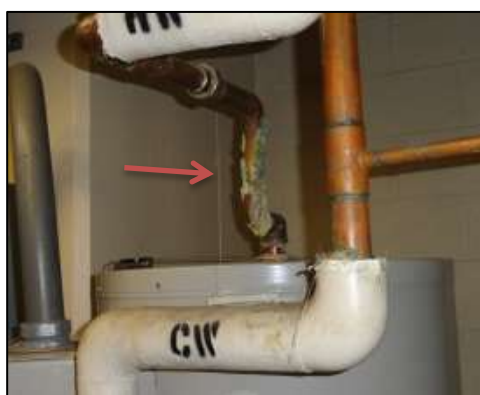
Figure 39: Possible corroding pipes on water heater at the Seventh District Station
