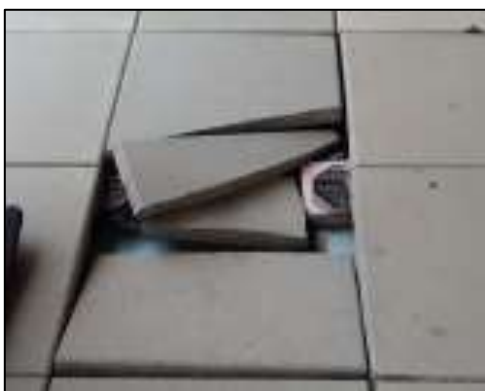
Figure 26: Example of broken walkway tiles at the Fifth District Station
