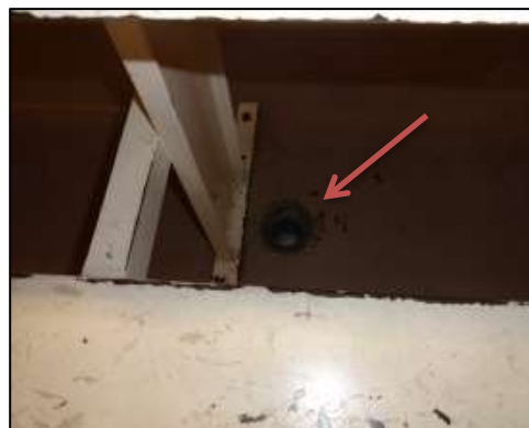
Figure 41: Drain cover missing in cell under table at the Seventh District Station
