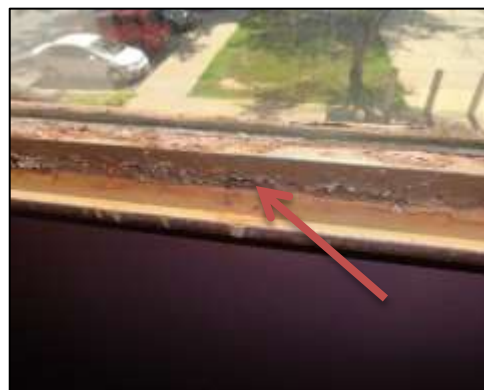
Figure 11: Figure 12: Peeling paint/rust on window sill at Second District Station
