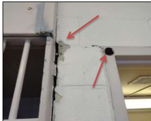
Figure 15: Holes and cracks by holding cells at the Third District Station
