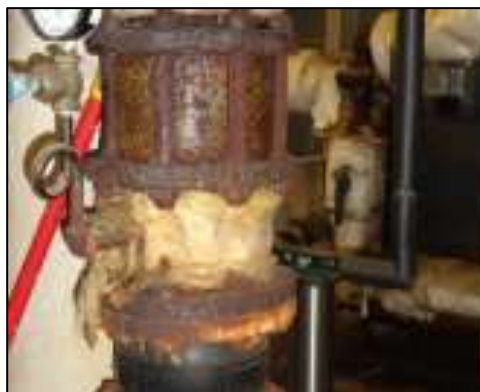
Figure 38: Example of corroded equipment in boiler room at the Seventh District Station
