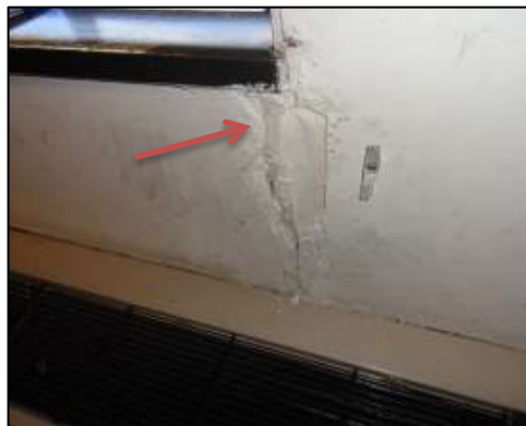
Figure 18: Water damage under window sill at the Third District Station
