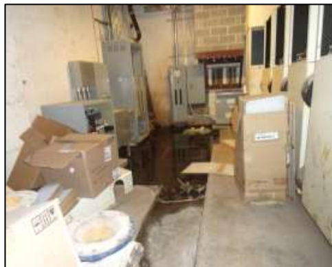
Figure 7: Example 2 of leak in boiler room in First District Station
