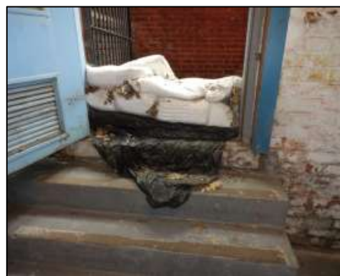
Figure 9: Sandbags outside exterior boiler room door of the First District Substation
